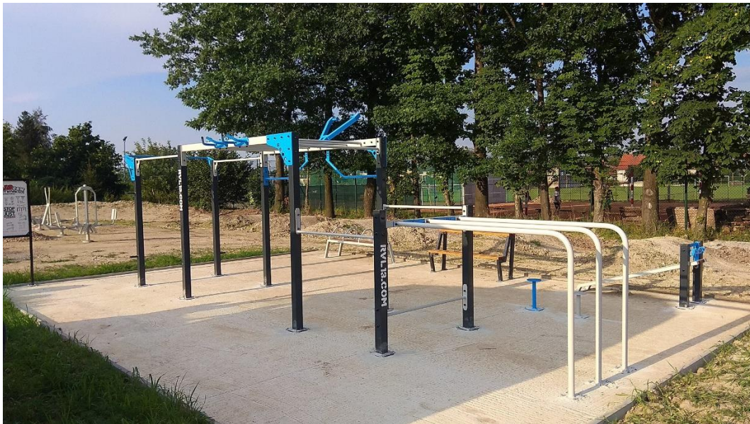
Concrete slab prepared for Liquid EPDM
