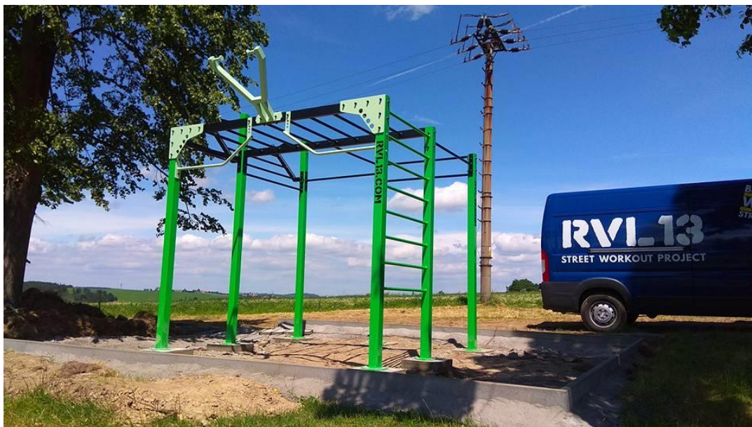
Concrete footings - ready for loose mat.
