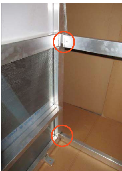
c) Stick plate into rear wall profile
